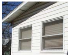
Siding and Windows BEFORE
