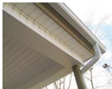
Soffit and Fascia AFTER
