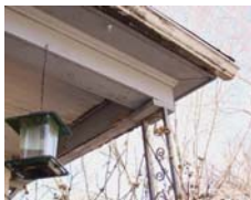
Soffit and Fascia BEFORE
