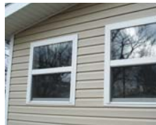
Siding and Windows AFTER
