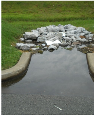
Trash at the drainage ditch inlet that the curb and gutter lead to.
